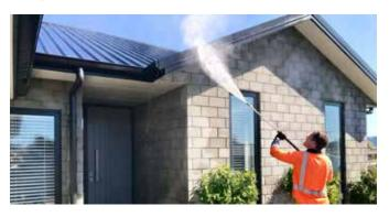
The 0° nozzle is the highest-pressure nozzle and emits a pencil jet of water that should only be used for precision industrial cleaning. This nozzle is typically used to remove tar, glues, rust, resins and barnacles and can damage the substrate and cause harm if used incorrectly.
